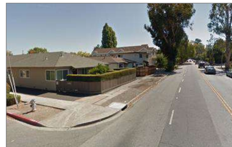
Non-compliant curb ramps
